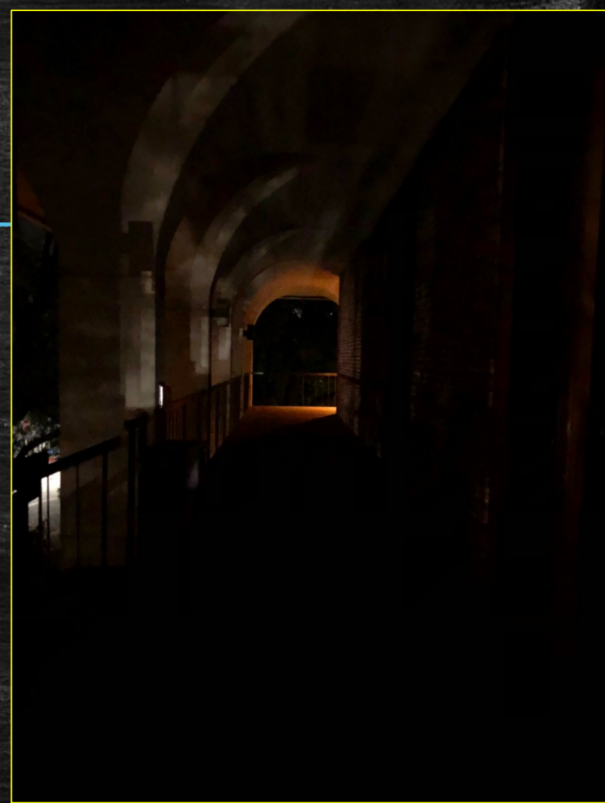
Photo showing lack of lighting on second floor Emeritus Photo by Rafael Vasquez
